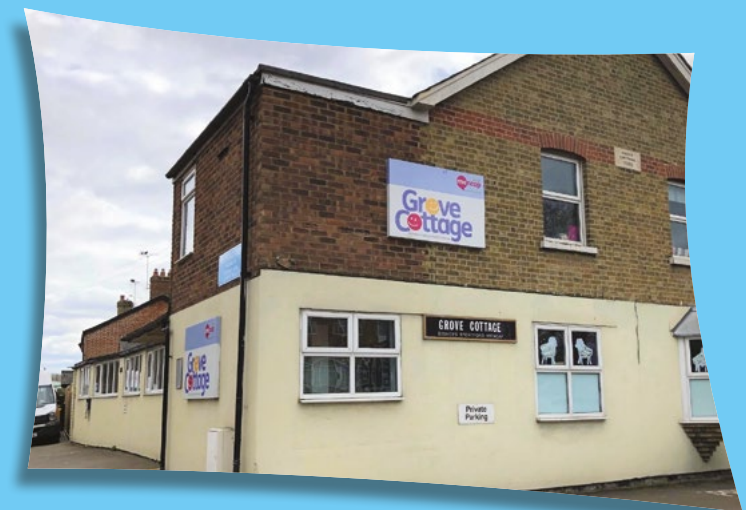
Our current Grove Cottage building
